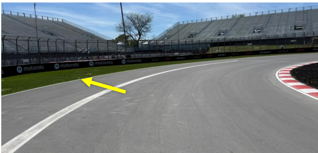
Pit Exit (arrow position corrected)
