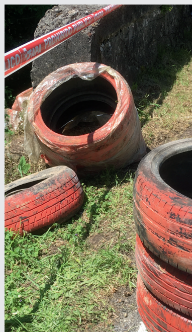
Poorly positioned and constructed tyre stack
