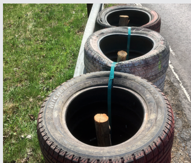
Tyre stack well constructed
