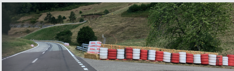
Good use of bales and connected tyres to protect competitors.
