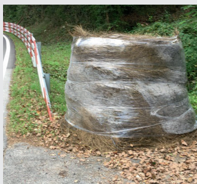
Guardrail nose not protected
