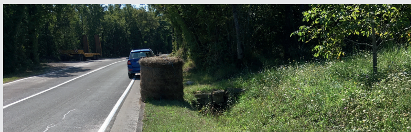
Concrete drain not protected
