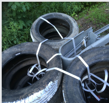
Poorly constructed tyre stack
