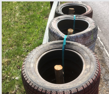
Tyre stack well constructed
