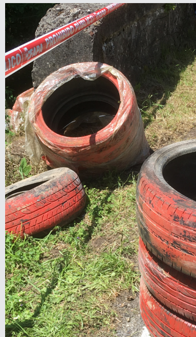
Poorly positioned and constructed tyre stack
