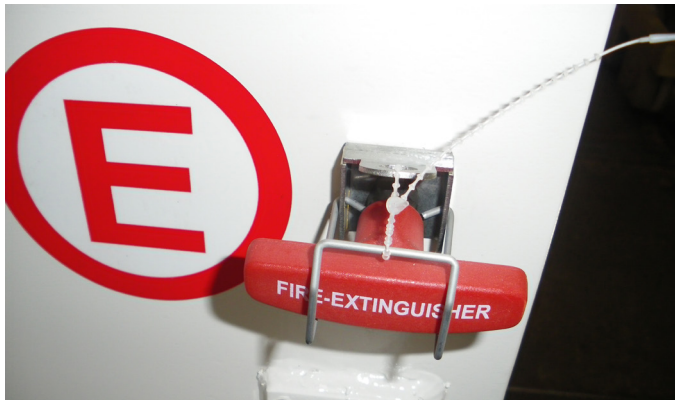
Figure 28. Label "E" and seal on the handle
