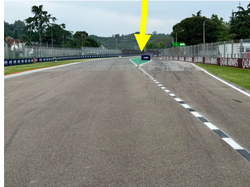
Figure 3 Bollard at Pit Entry
