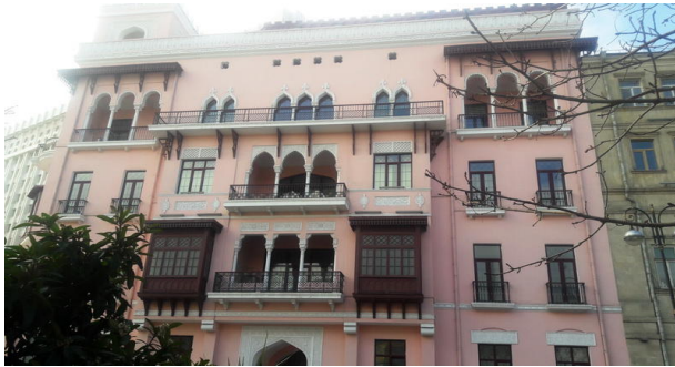
Building 5: 25, Istiglaliyyat Street. 3 rd floor balcony, facing Philharmonic.
