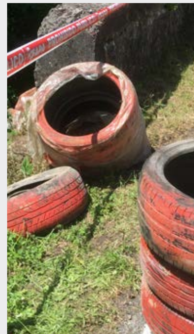
Poorly positioned and constructed tyre stack
