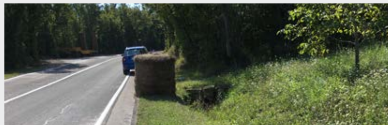
Concrete drain not protected
