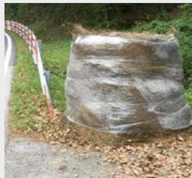
Guardrail nose not protected
