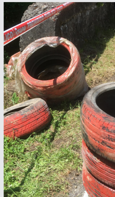
Poorly positioned and constructed tyre stack
