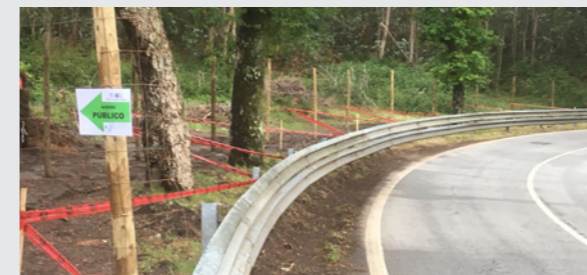
Good tape and temporary fencing to keep spectators at a safer distance
